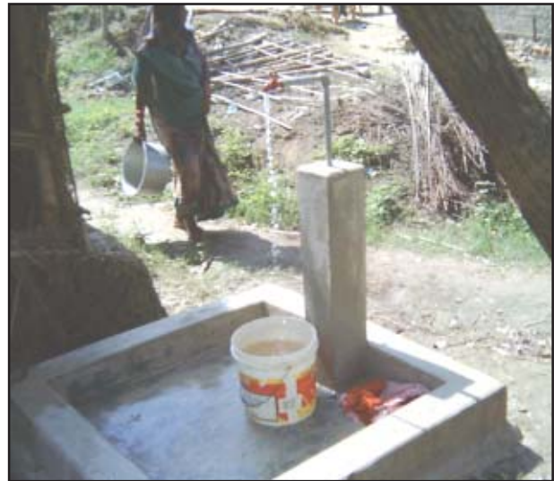
Community Tap for Potable Water
